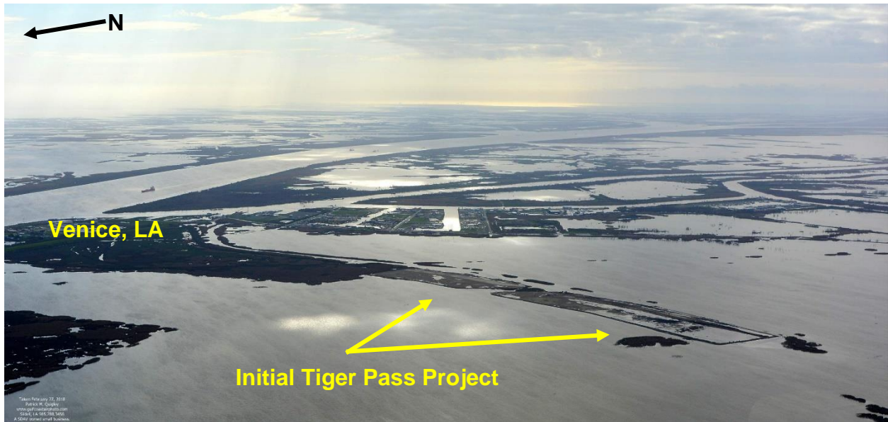
Figure 5. Late Stage Construction of Initial LCA BUDMAT at Tiger Pass Project in Vicinity of Venice, LA.
